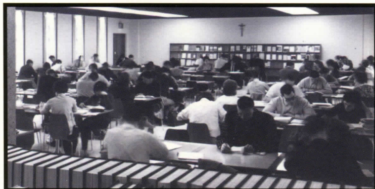
The Shannon Library Reading Room, 1964
